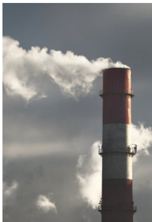
TotalEnergies aims to be carbon neutral by 2050.
