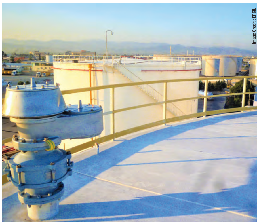
Recent incidents prove that specially configured tank equipment such as the pressure / vacuum relief valve with flame arrester minimises the risk to almost zero in storage tank refineries.
