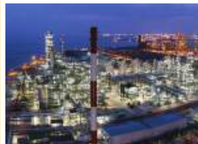
Orange Business Services works with major petrochemical and gas companies in Saudi Arabia
