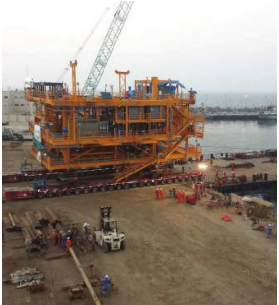
The Jalilah B topside being loaded out in Lamprell's Sharjah yard in late September
