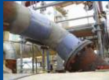
Composite Repairs
